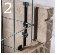
Use connector to attach Tandem Veneers to grid
